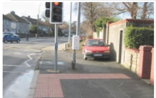
Tactile paving slabs
