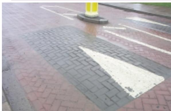
Bitumen based material with block pattern
