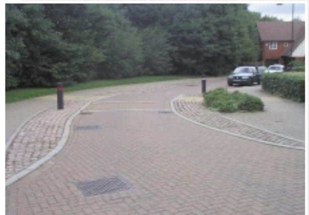
Bends in the road reduce excessive forward visibility and control speed on new roads
