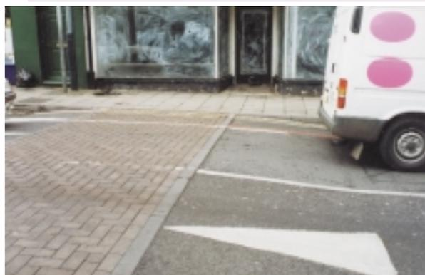
Ramp with composite construction and 'lip' between materials
