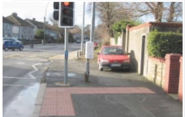
Tactile paving slabs
