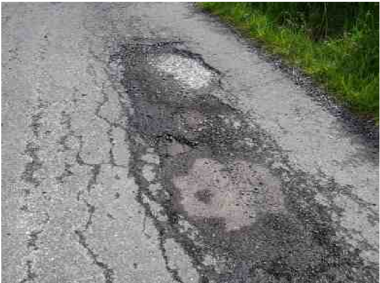
Very Poor/failed Patching with potholes and structural distress evident.
