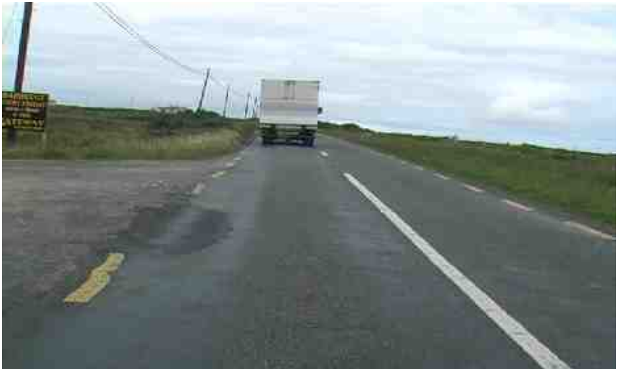
Rating 4: Edge problems, rutting, out of shape and other defects present.
