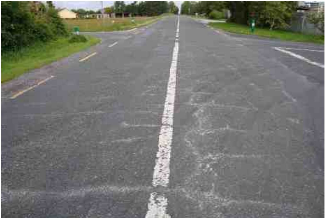
Combined Transverse and Longitudinal cracking.
