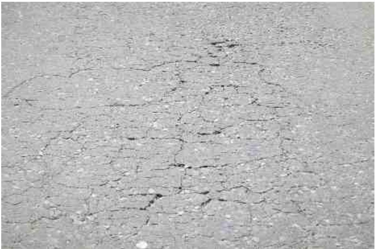
Wide area of alligator cracking.
