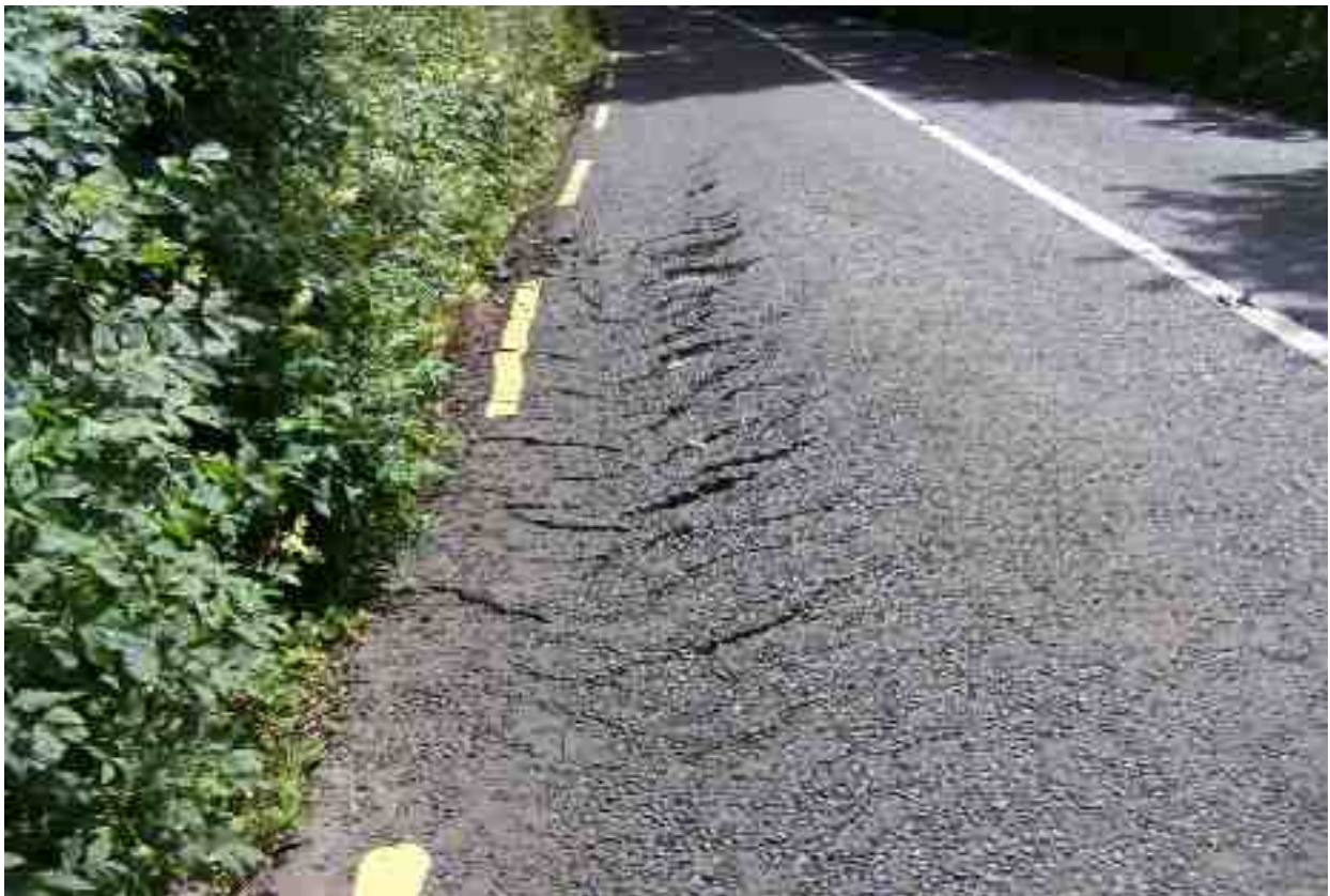
Slippage cracking with underlying stability problems.
