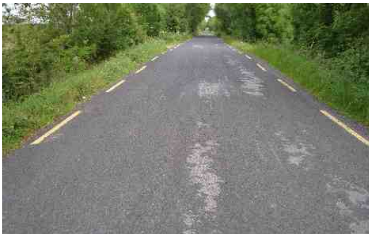
Rating 6: Pavement surface distortion requiring reduction in driver speed, surface defects also present.
