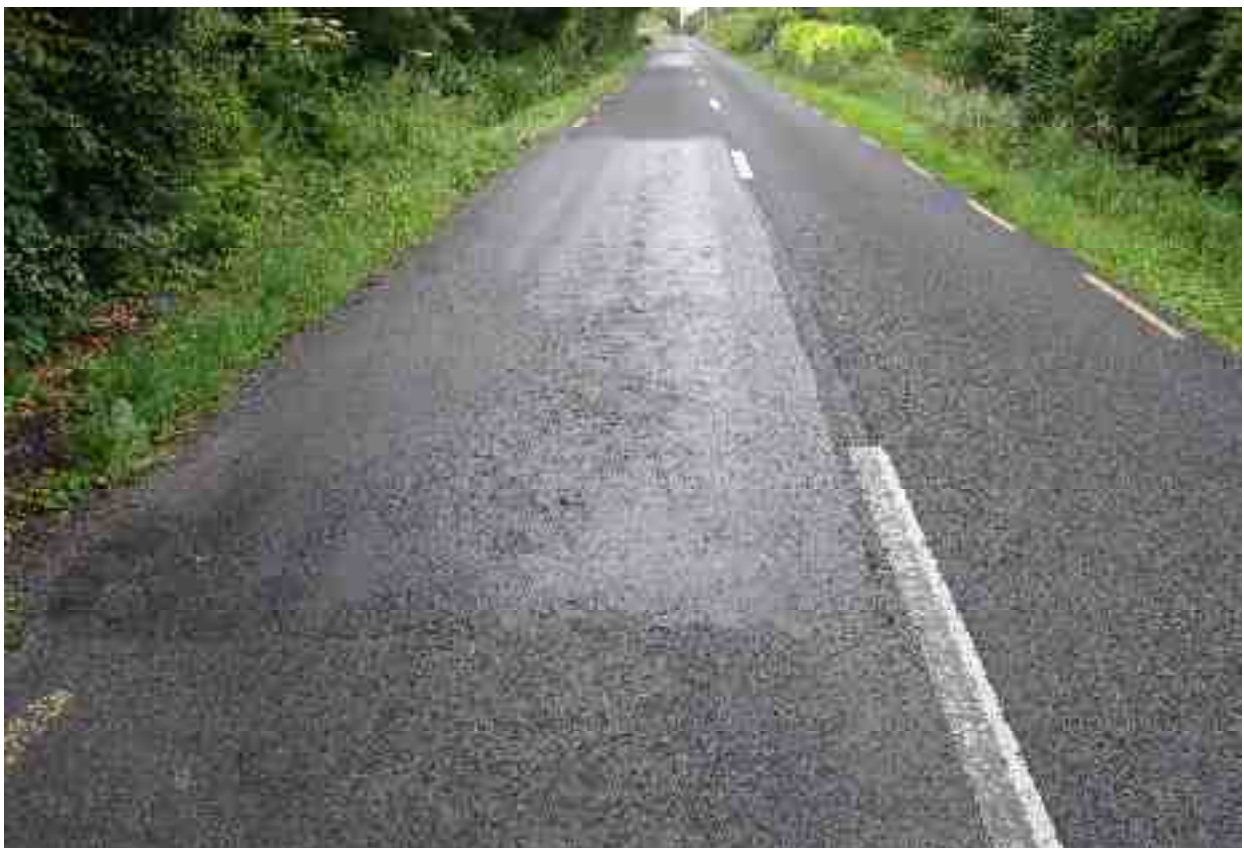
Large patching in reasonably good condition.
