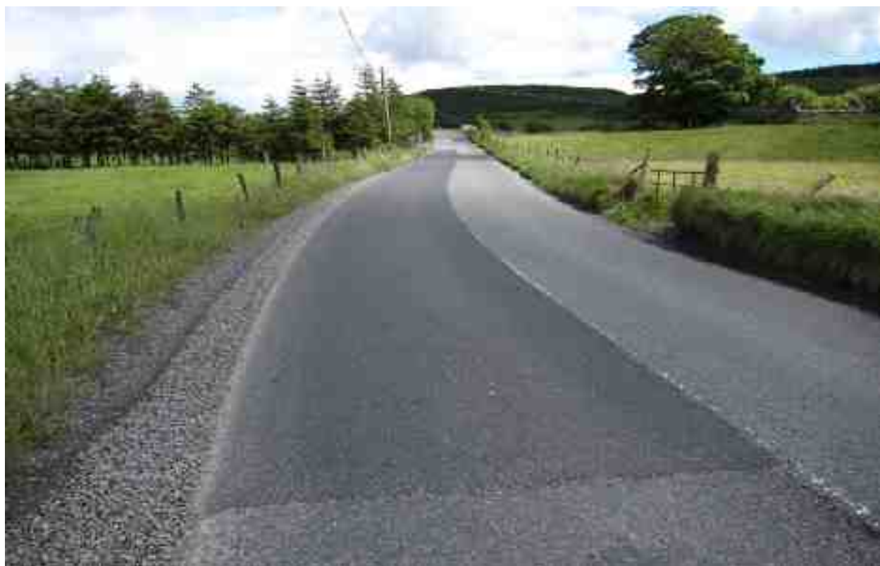
Rating 9: Road recently surfaced, good shape, little or no visible distresses.
