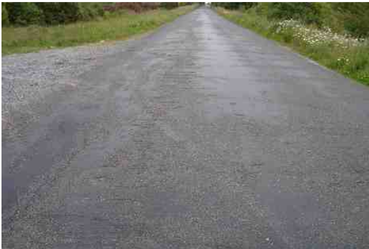
Rating 6: Transverse cracking, weak support.
