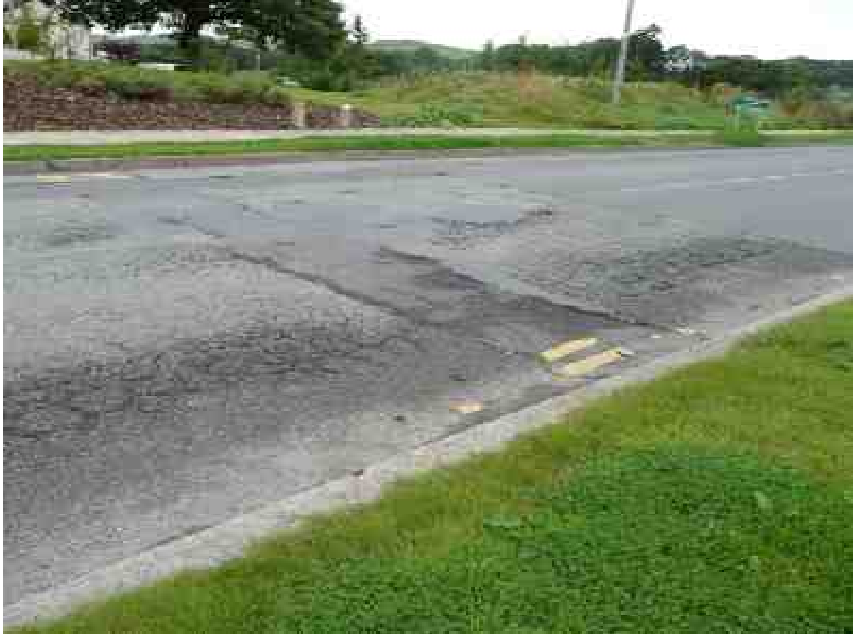
Extensive patching in very poor condition.
