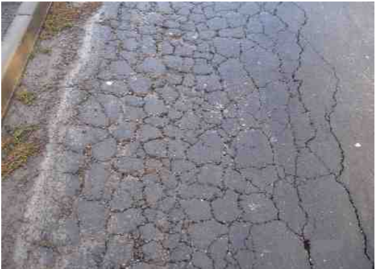
Characteristic “Chicken wire” crack pattern shows smaller pavement pieces and patching.
