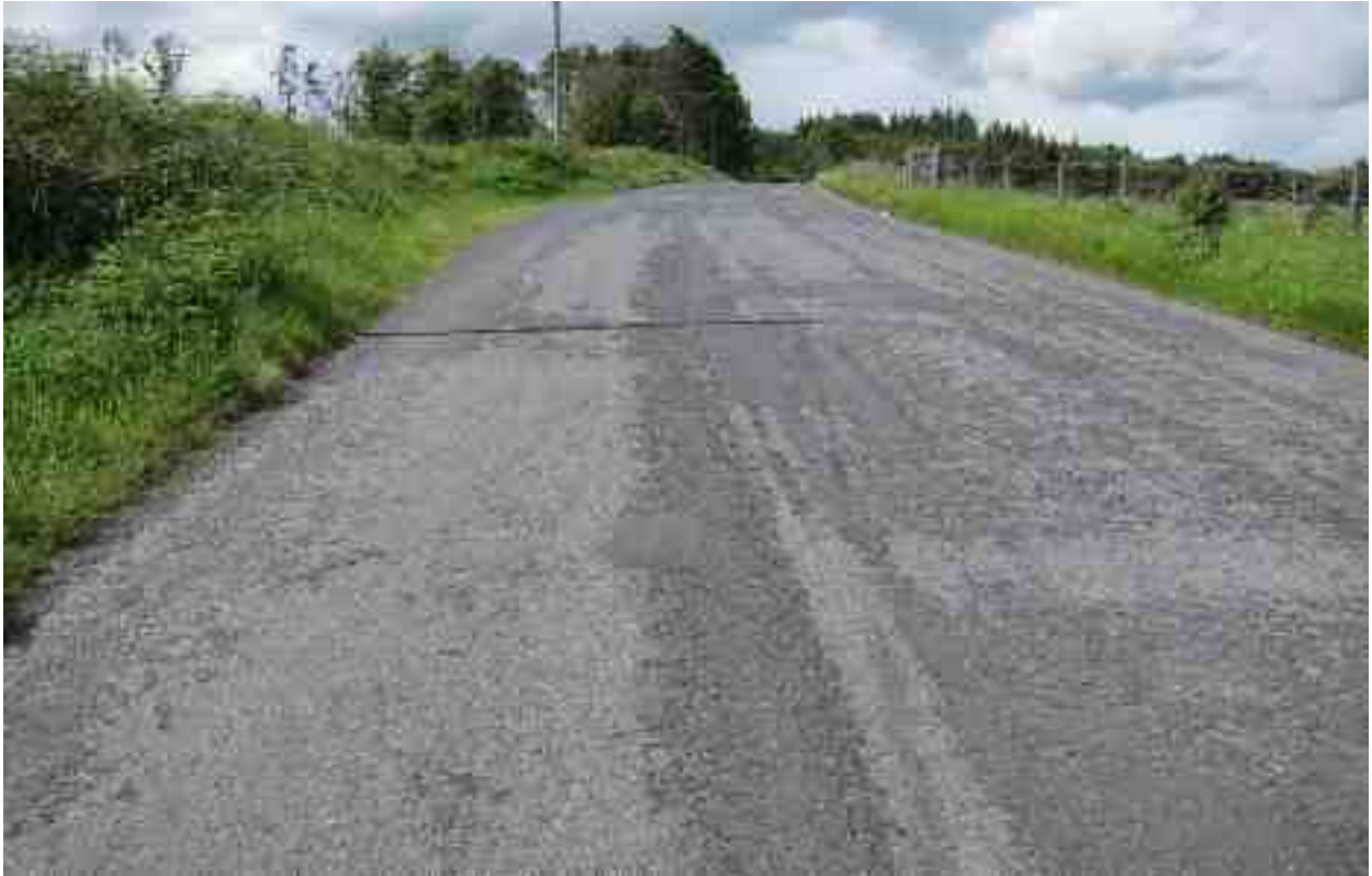
Rating 7: Extensive Ravelling (> 30%) over most of pavement surface.
