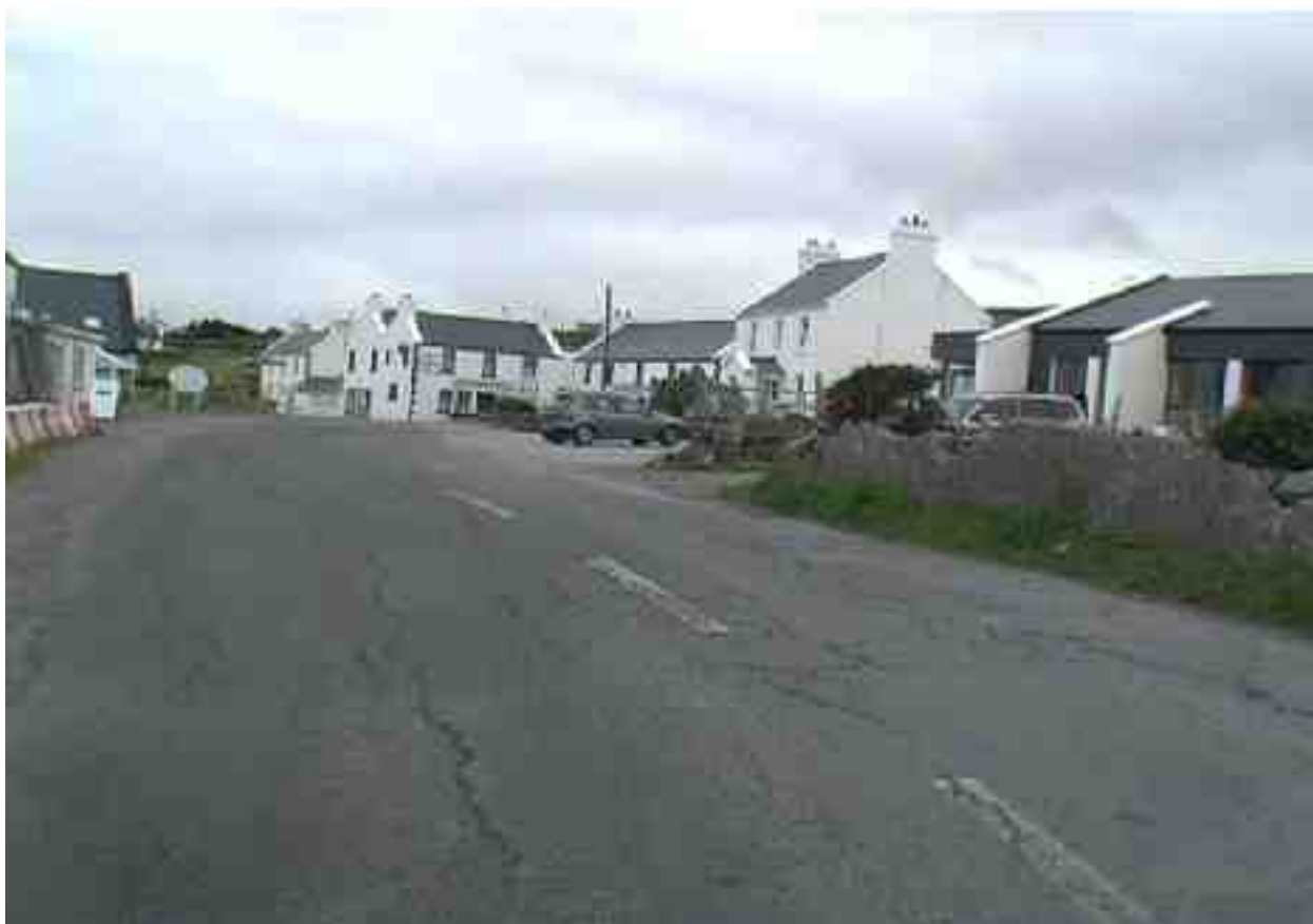
Rating 3: Significant alligator cracking and structural problems over large areas.
