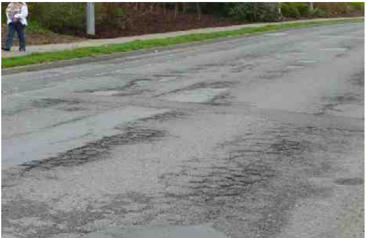
Rating 3: Extensive alligator cracking and structural distress.
