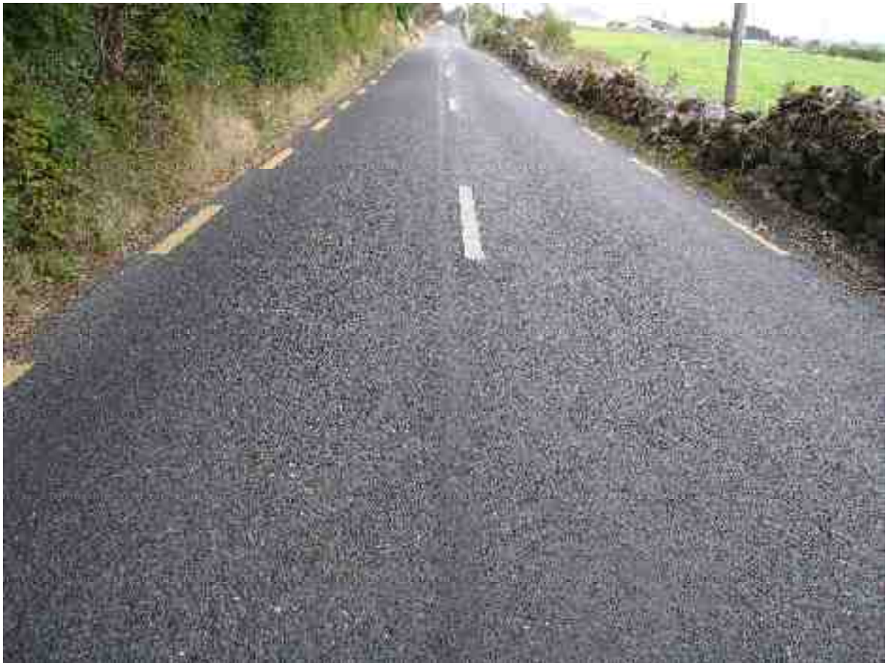
Rating 9: Recent surface dressing with some minor bleeding.
