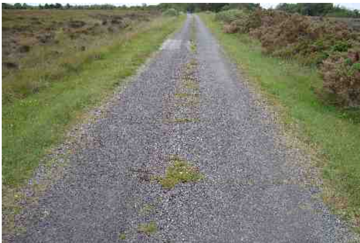
Rating 6: Old surface, surface seal is clearly broken due to transverse cracking, moisture can penetrate the surface. Road in need of surface restoration to restore shape and waterproofing surface layer.
