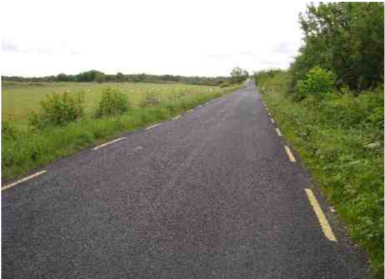
Surface deformation and shape problems (note road marking on left edge for reference).
