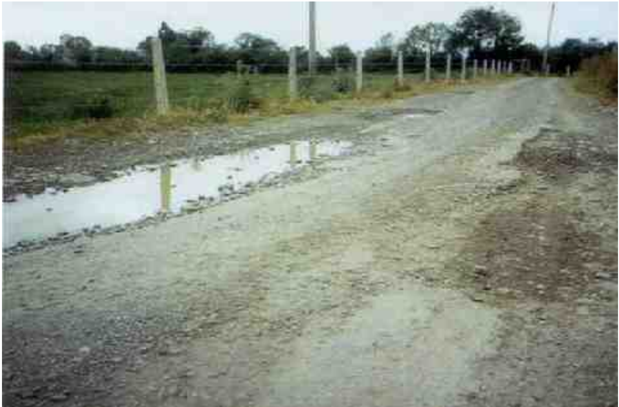
Road not passable by vehicles at speeds above walking pace. Damage to vehicle may occur.
