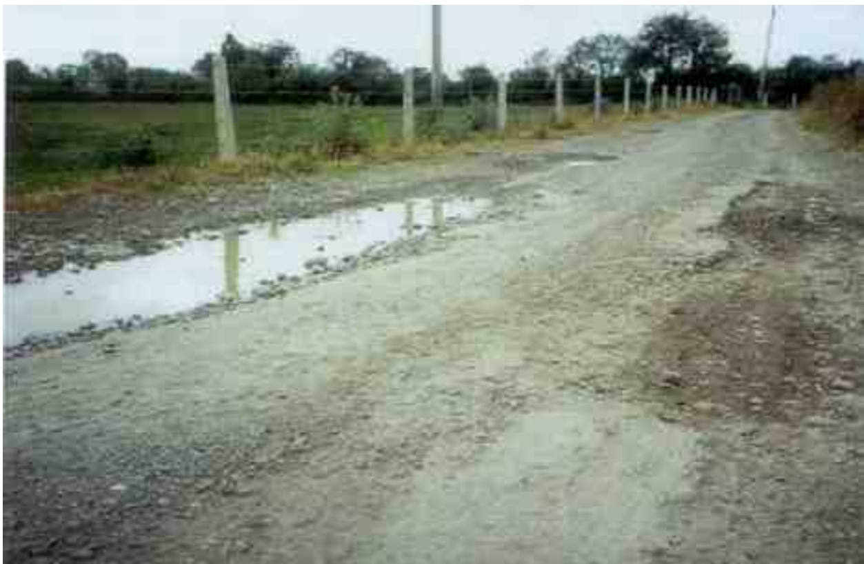
Rating 1: Road surface disintegrated, extensive road failure.
