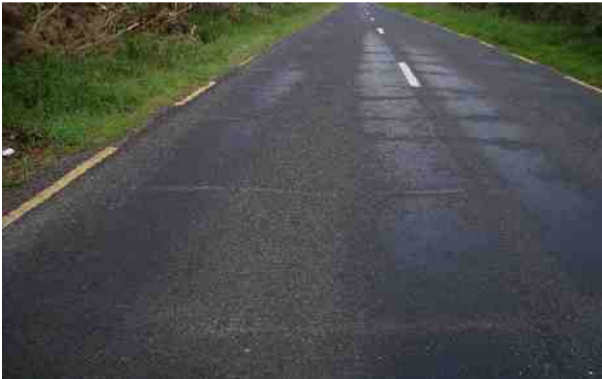
Rating 6: Pavement surface distortion, transverse cracking at regular intervals.
