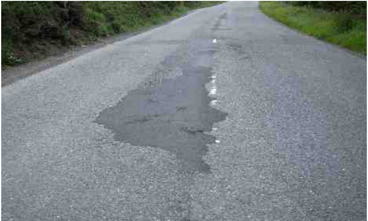
Rating 5: Loss of Shape, localised repair needed, patching in fair condition.
