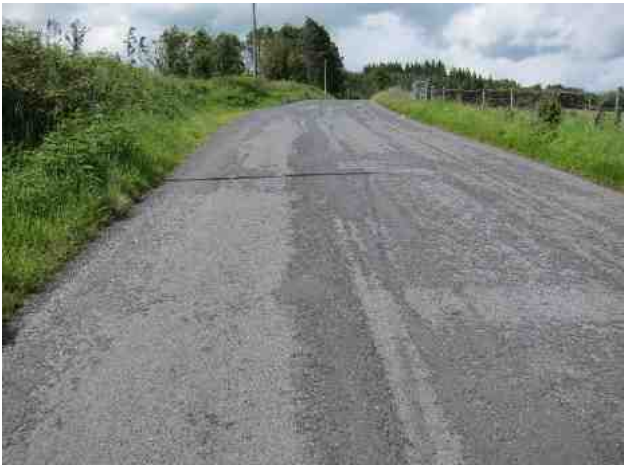
Severe Ravelling. Most of the new surface has been lost, exposing the older surface beneath.
