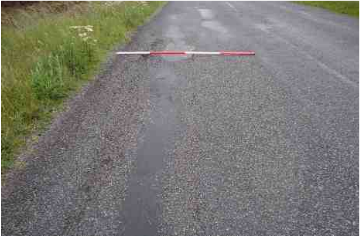
Severe Rutting over 50mm in depth evident in wheel path.
