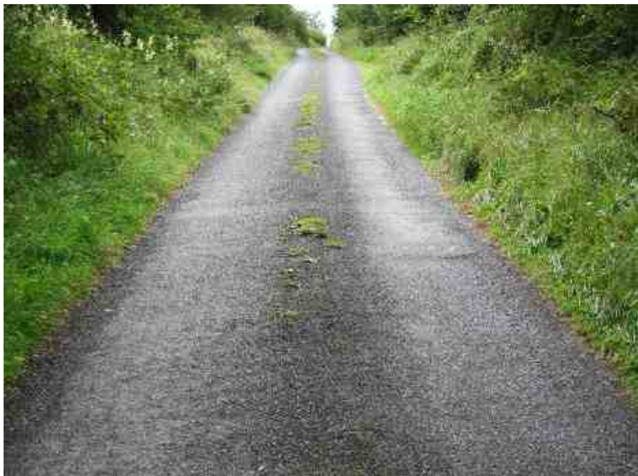
Rating 7: Old surface with some ravelling and aged appearance.
