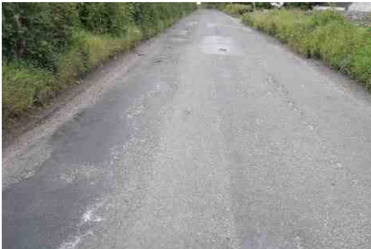
Rating 4: Alligator cracking, rutting, and potholes present.
