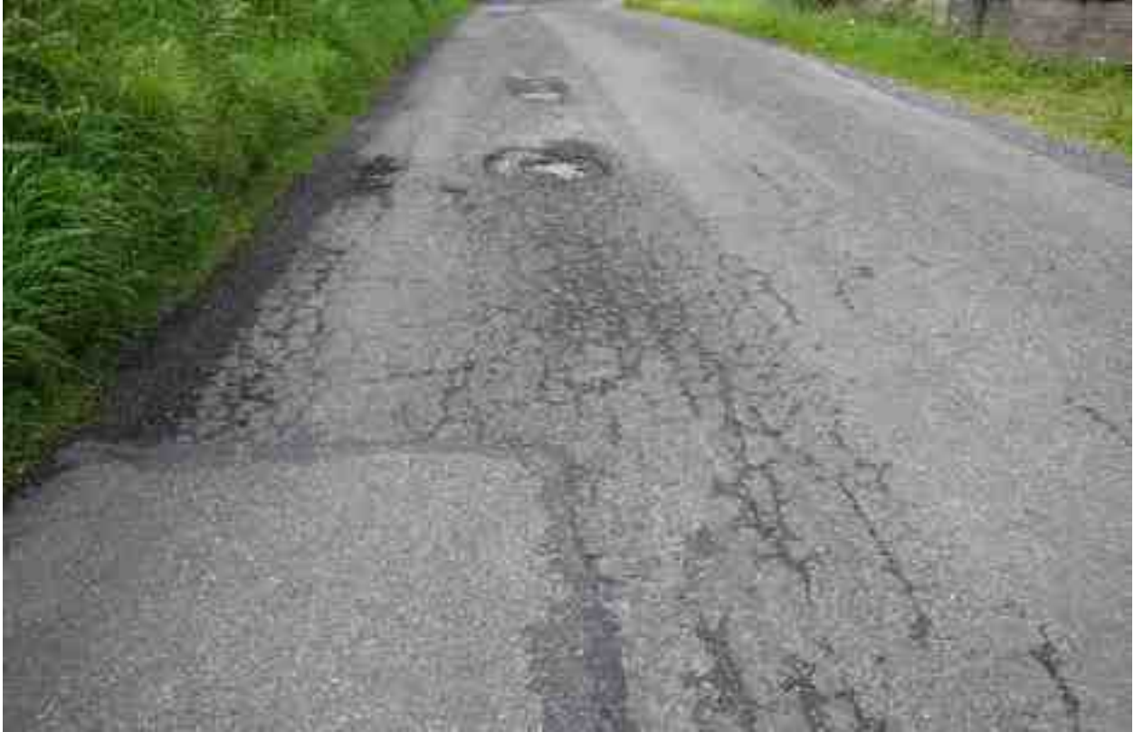
Rating 3: Significant alligator cracking over large areas, some potholes and edge problems.
