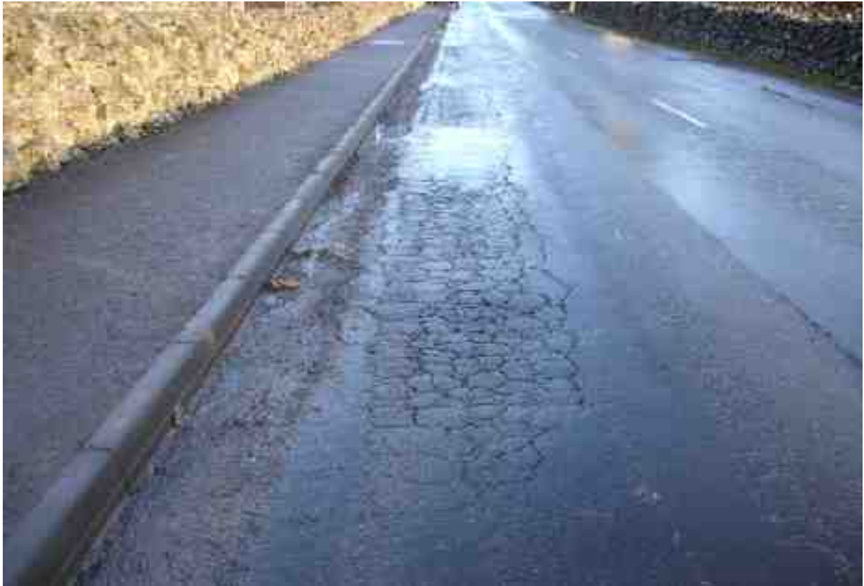
Open alligator cracking with settlement along lane edge most likely due to very weak subgrade.
