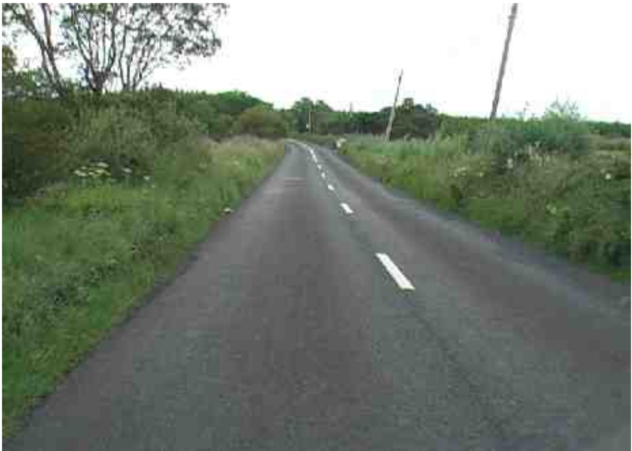
Edge breakup/cracking and material loss from weakened subbase and traffic loads.
