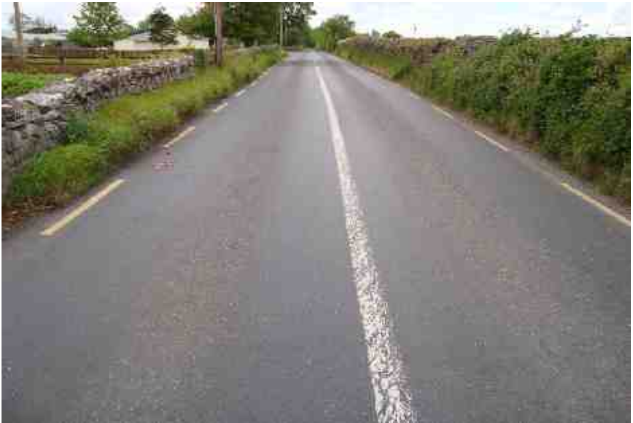
Rating 7: Bleeding on greater than 30% of pavement surface.
