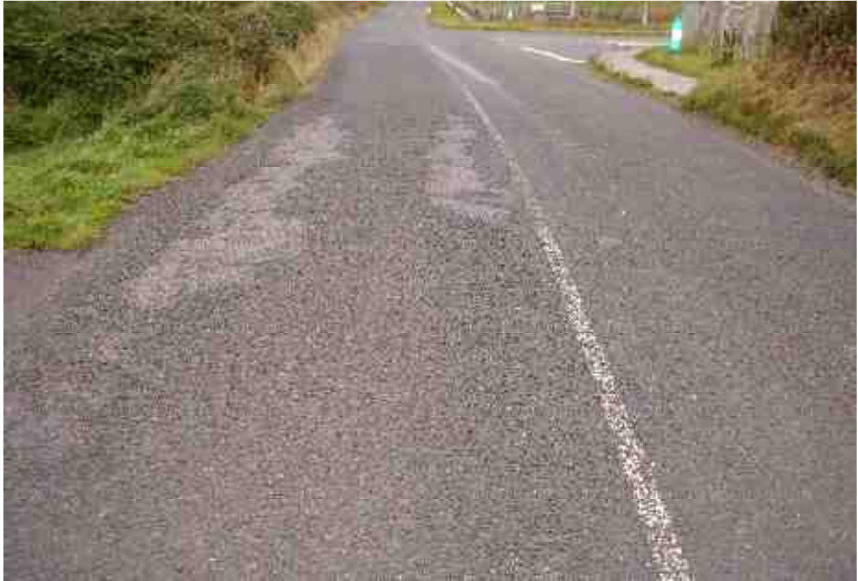
Moderate Ravelling evident in wheelpaths.
