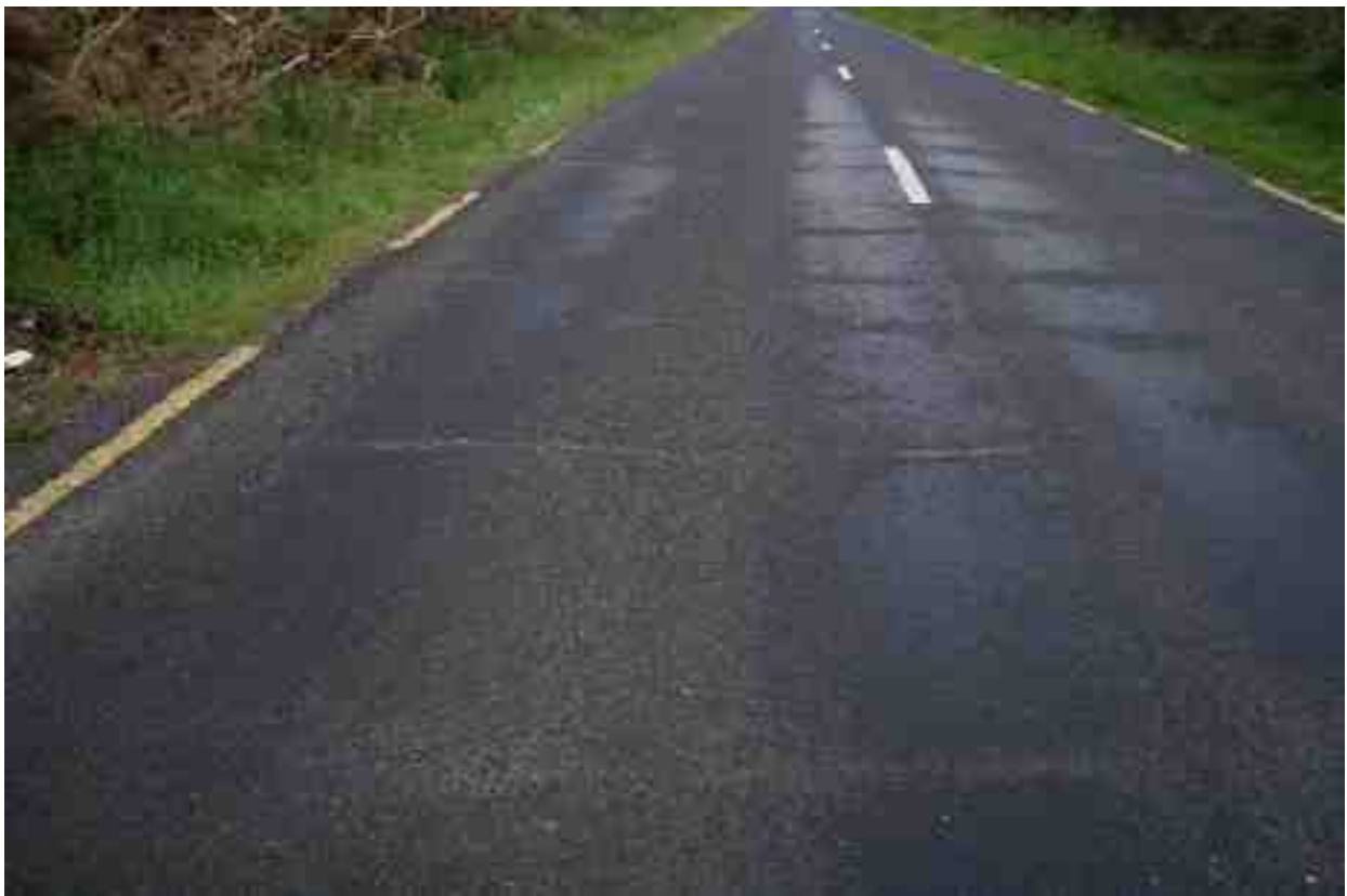
Regular pattern of transverse cracking – bleeding also evident in the wheelpaths.
