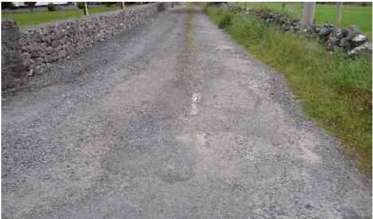
Rating 2: Failed areas, extensive patching in very poor condition, loss of surfacing in places.
