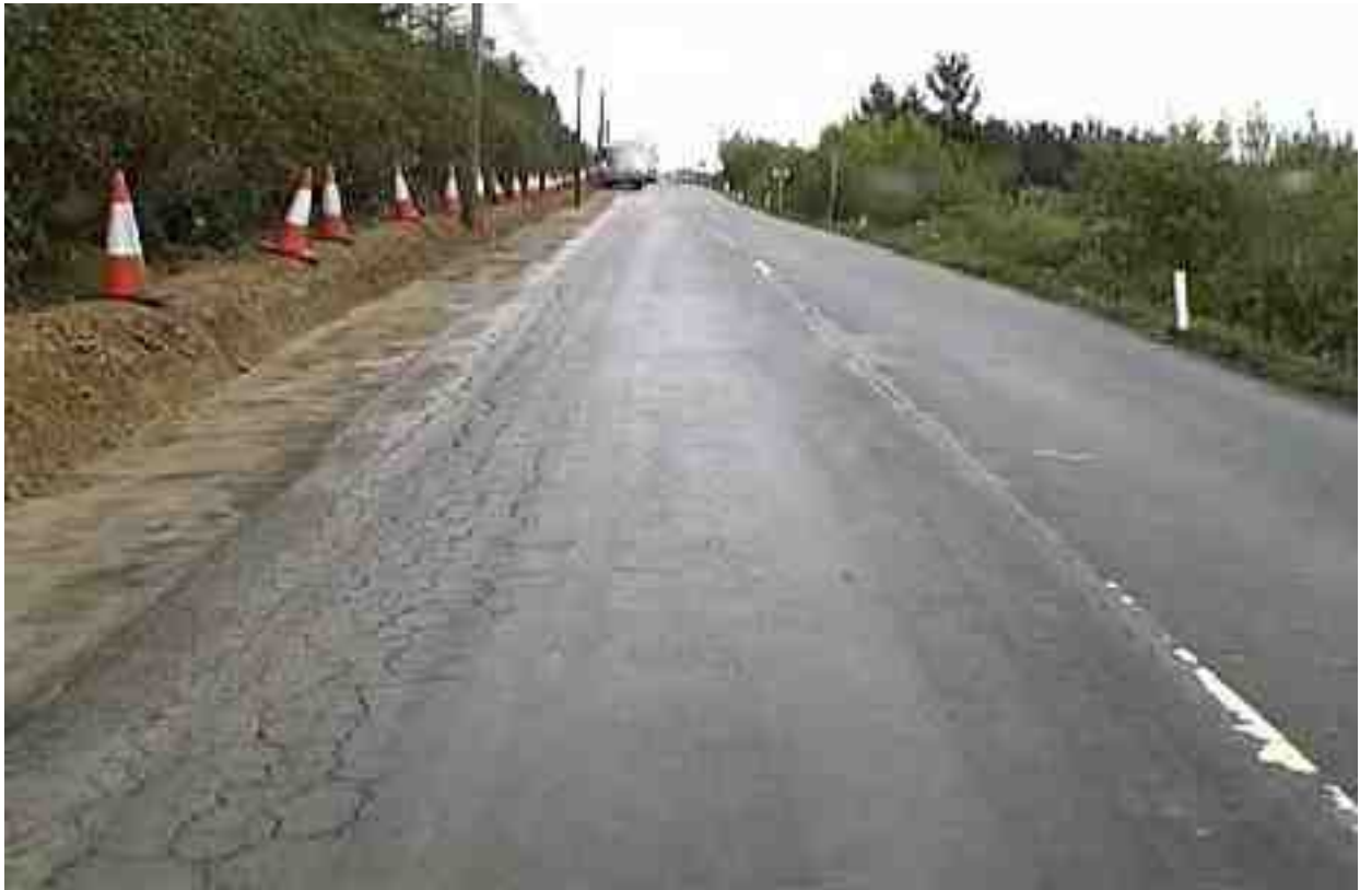
Multiple cracking within 300 mm of the pavement edge.
