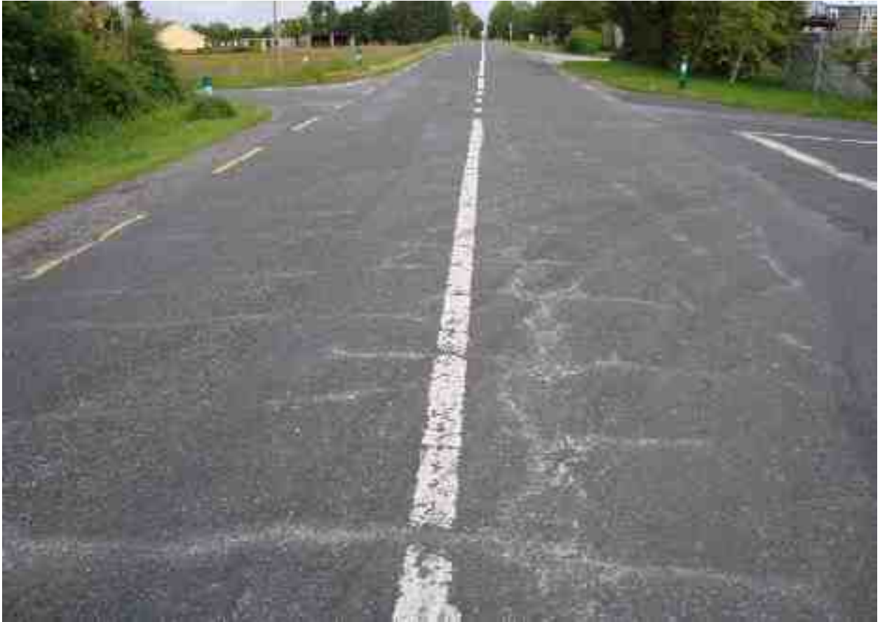
Rating 5: Extensive Longitudinal and Transverse Cracking, pumping of fines from under surface.
