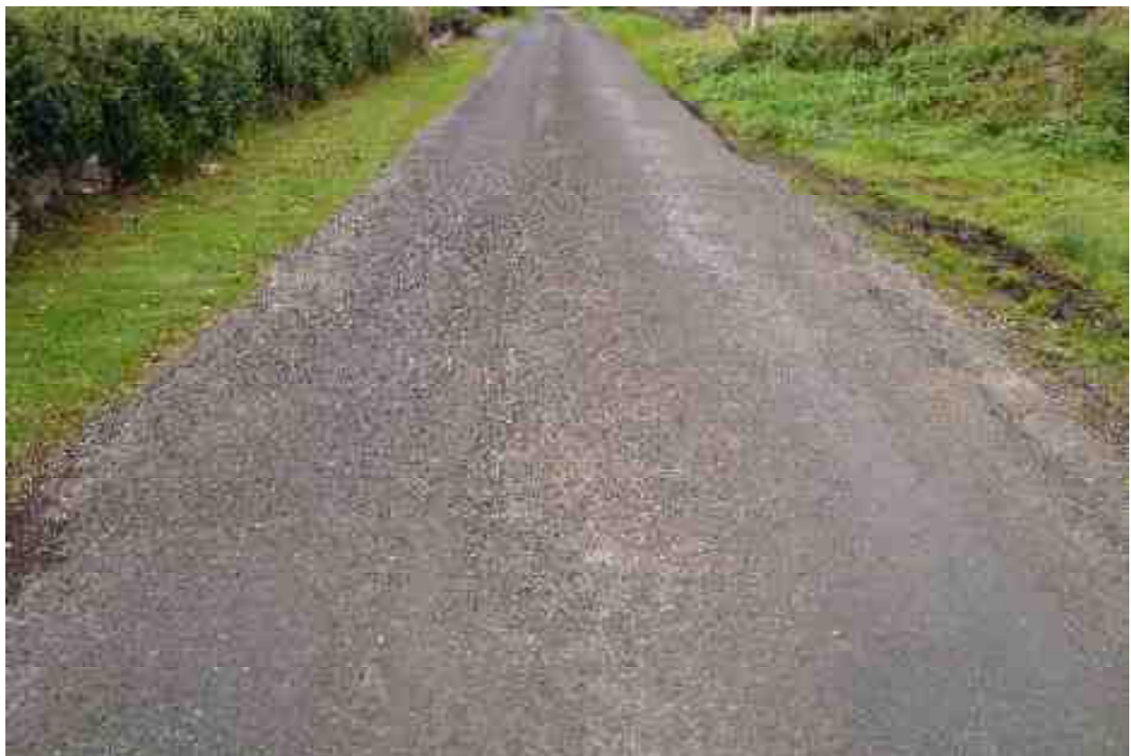
Rating 7: Old surface, Ravelling > 30% and aged appearance.
