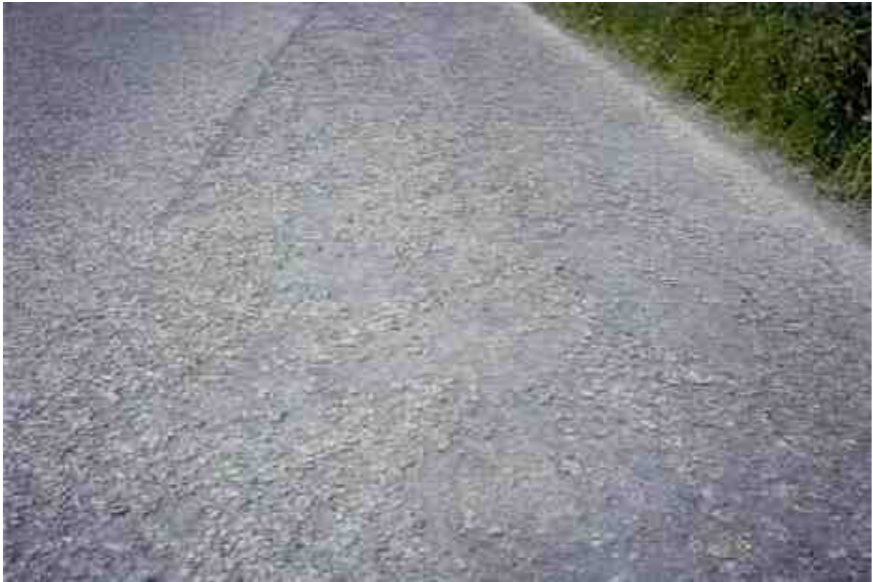
Moderate Ravelling. Small aggregate particles have worn away exposing tops of large aggregate.
