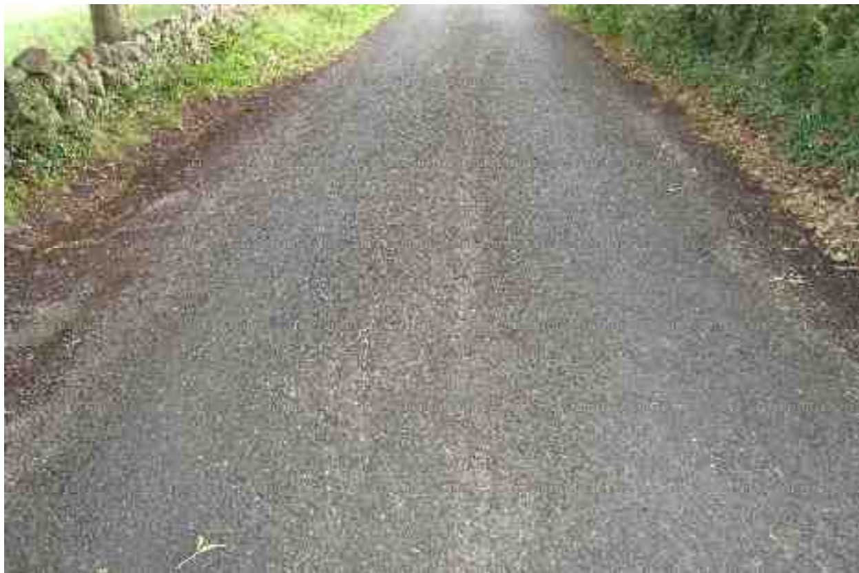
Rating 8: Ravelling, 10% to 30% of surface.
