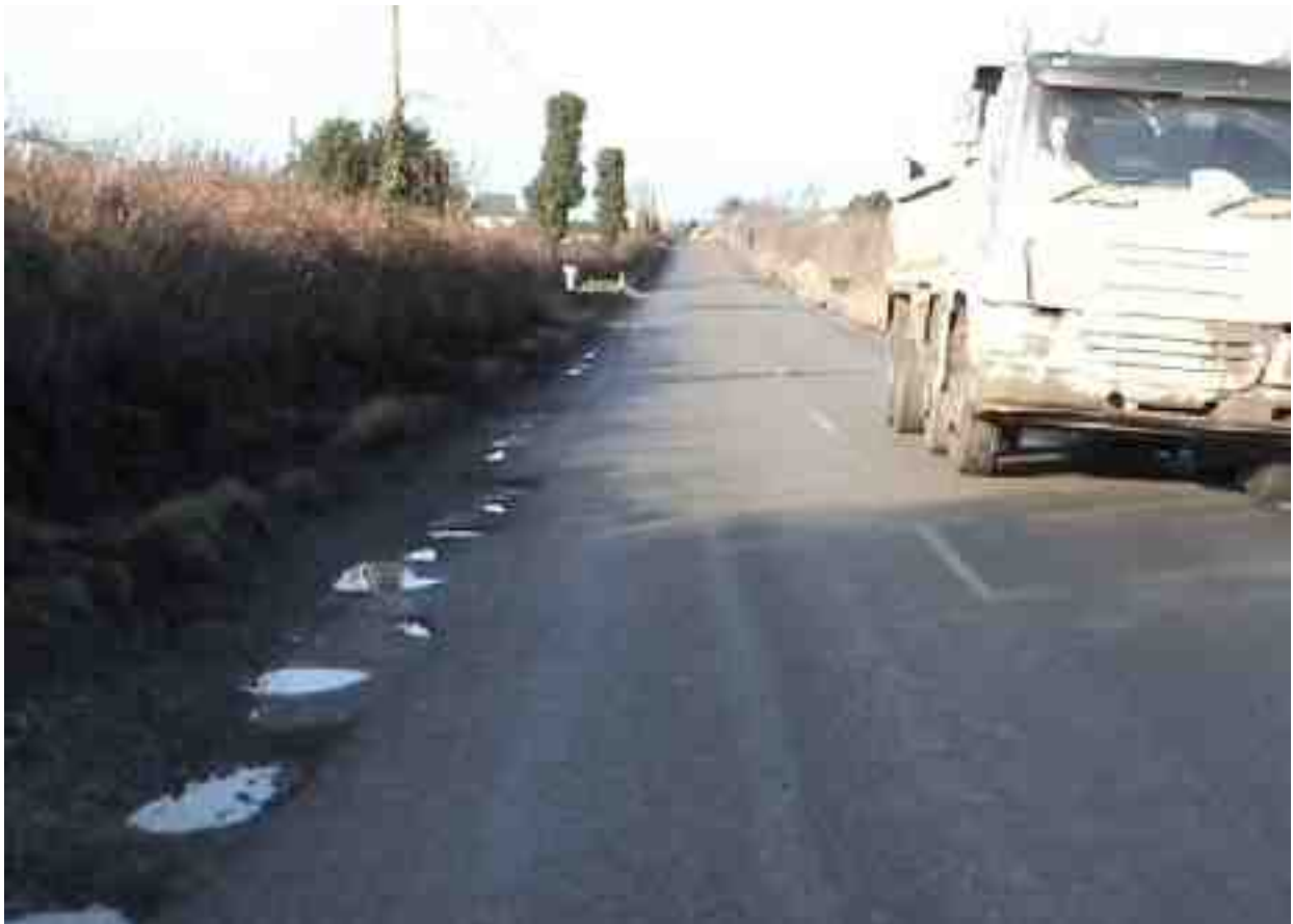
Potholes and loss of pavement material along the pavement edge.
