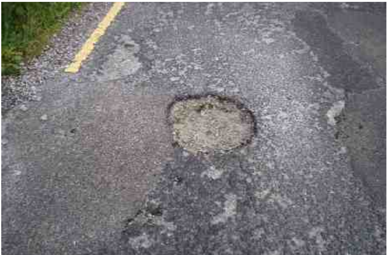
Reoccurring potholes due to poor patching work.
