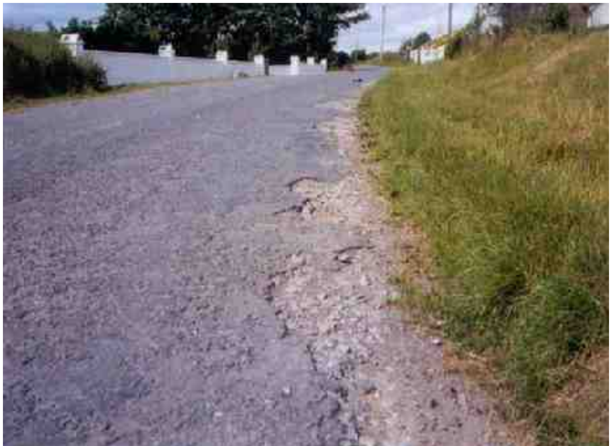
Loss of surface material at the edge of the road. This is ravelling, not edge breakup.
