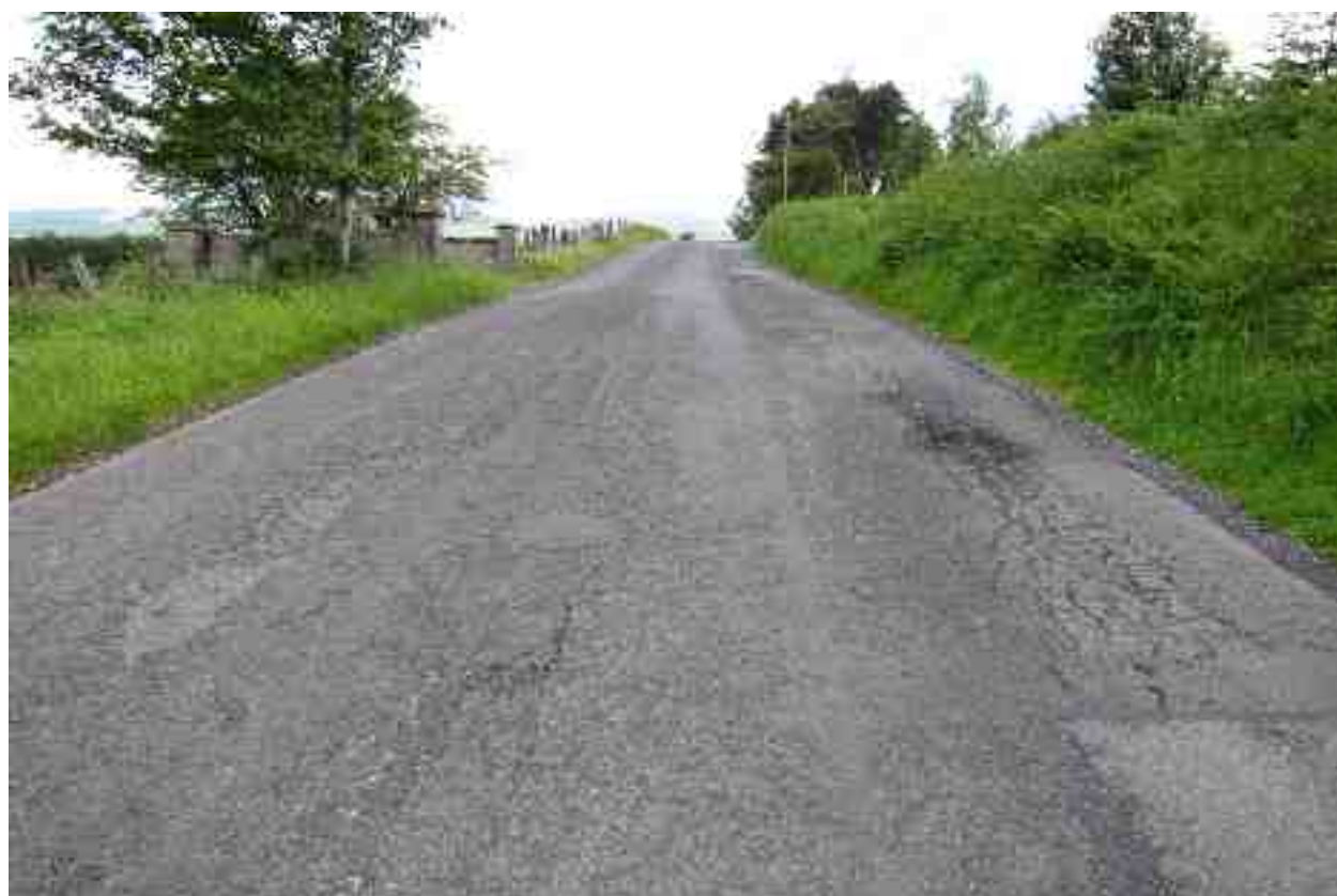
Rating 4: Alligator cracking, rutting and pothole formation in wheelpath. Structural distresses are clear.
