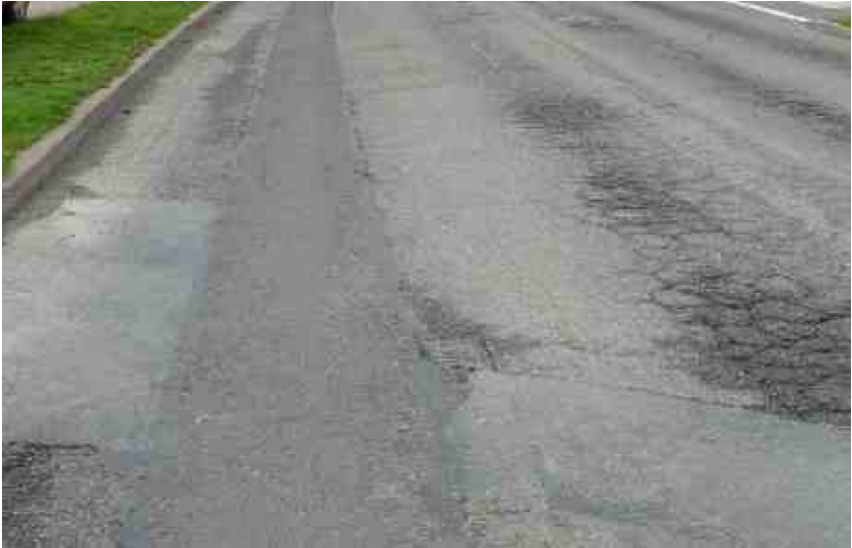
Typical patching repair of utility excavation.
