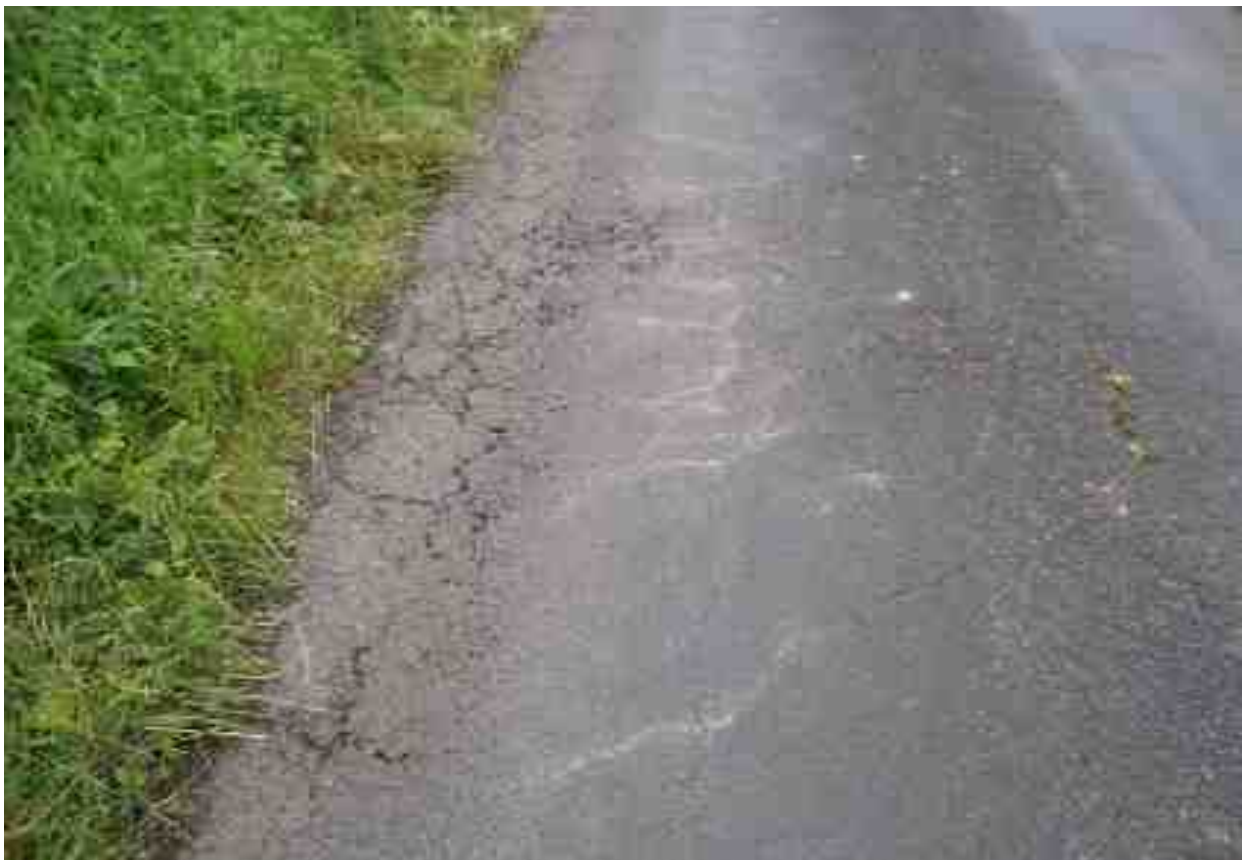
Edge Breakup identified by cracking at the edge of the road pavement.
