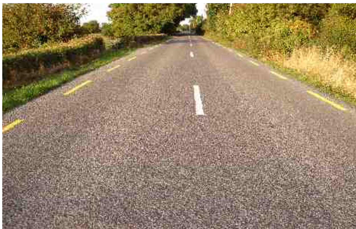
Rating 9: Road recently surfaced with some minor loss of chippings.
