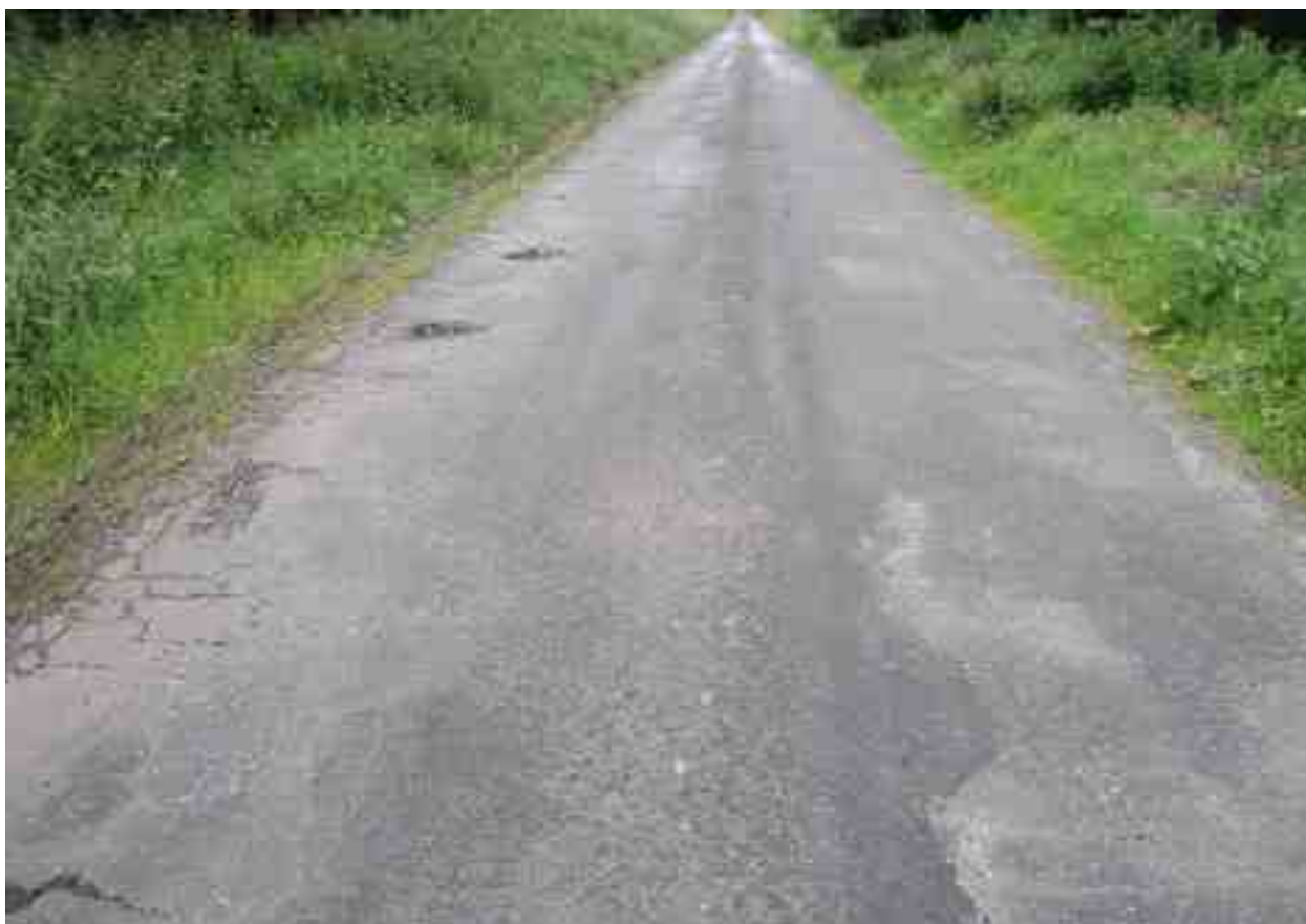
Rating 3: Edge problems/cracking, alligator cracking, rutting and potholes.
