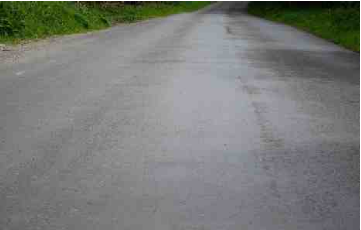
Rating 7: Extensive Bleeding (> 30%) over most of pavement surface.
