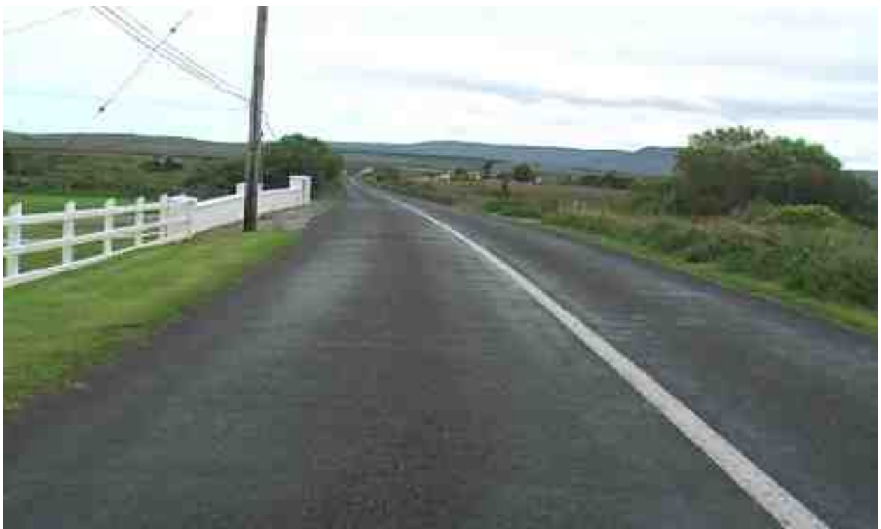
Rating 5: Surface distortion, transverse cracking, some localised structural distresses.
