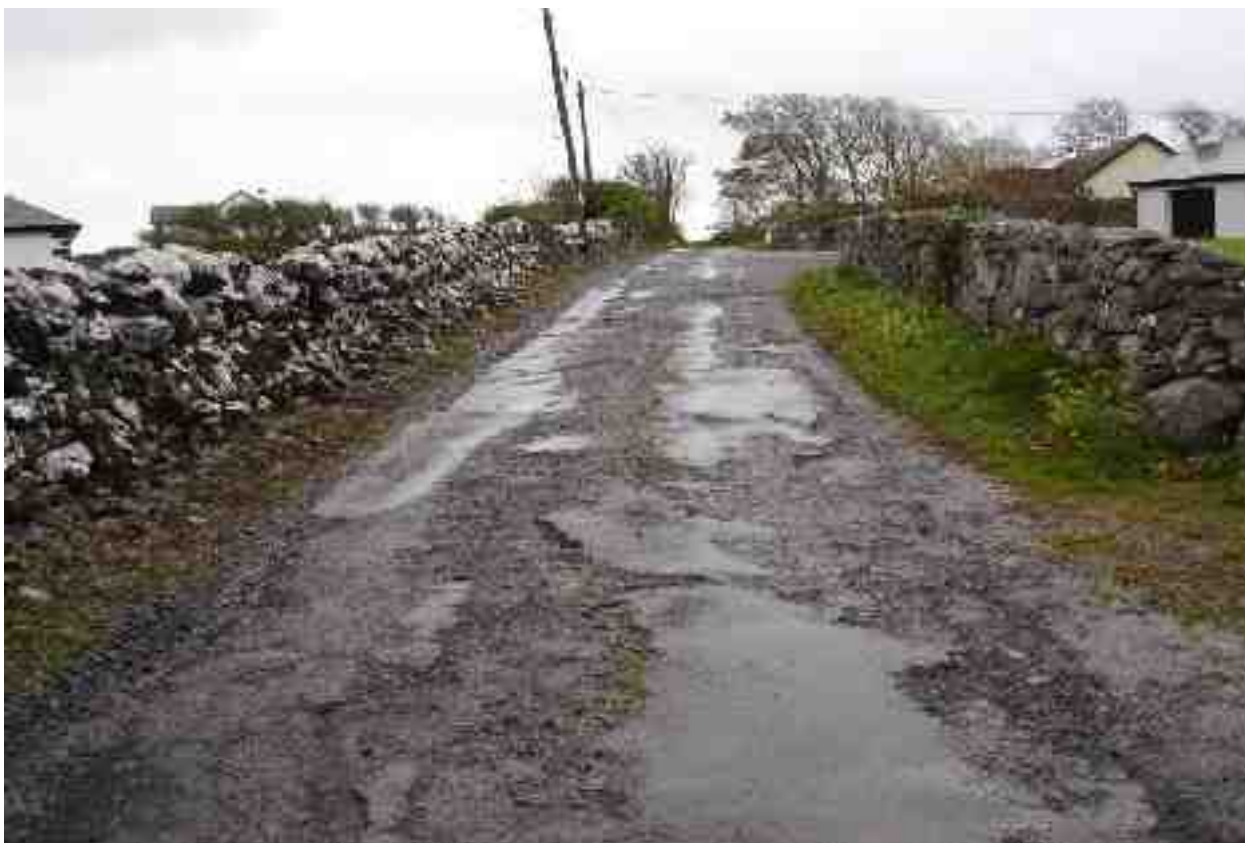
Rating 1: Significant loss of pavement surface, extensive road failure.
