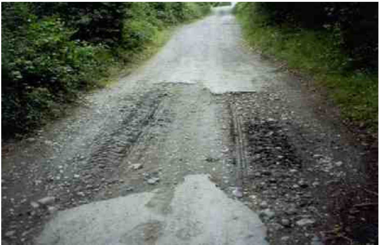
Disintegration of road resulting in exposure of subbase materials.
