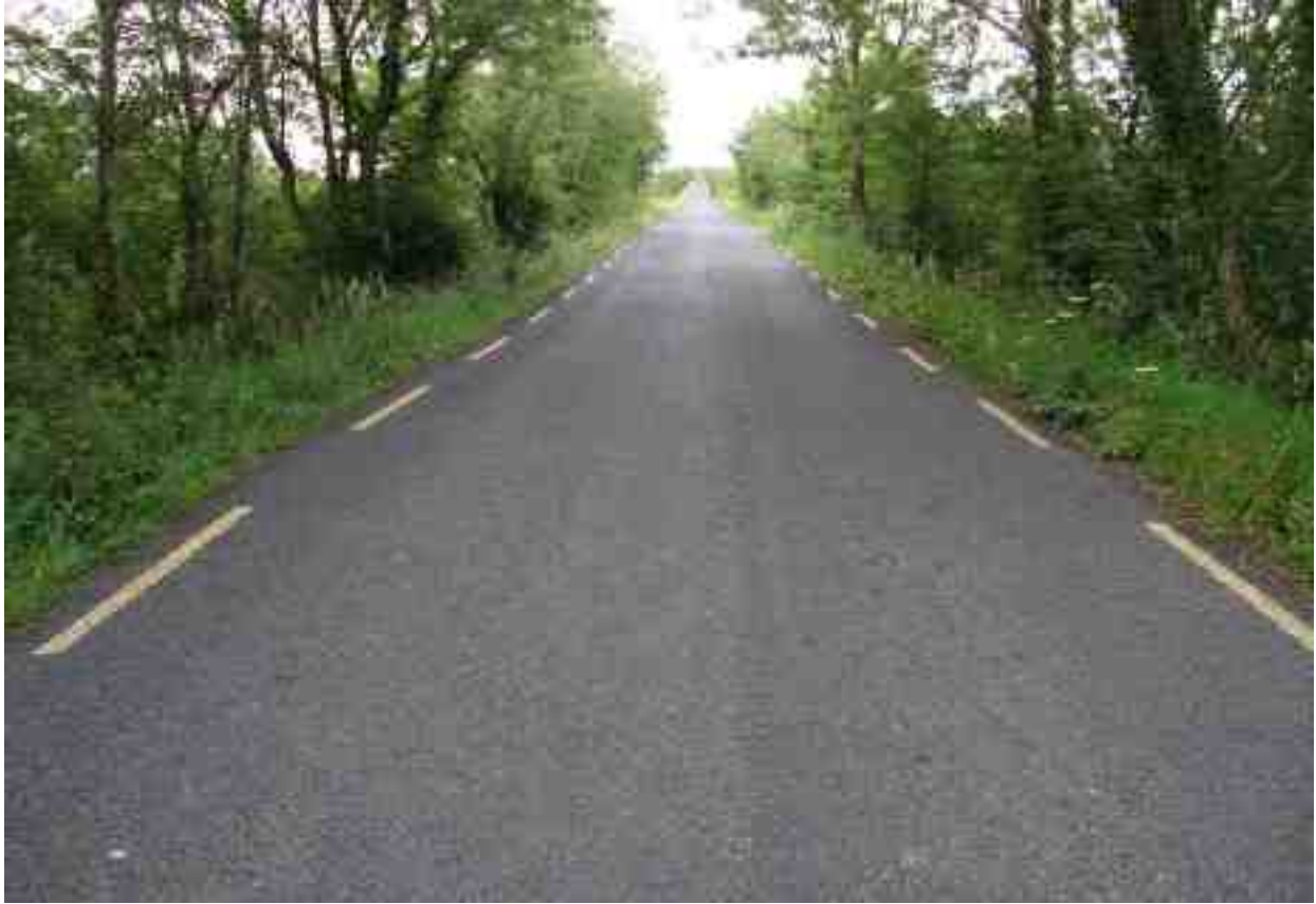
Surface Distortion (note road marking on left edge).
