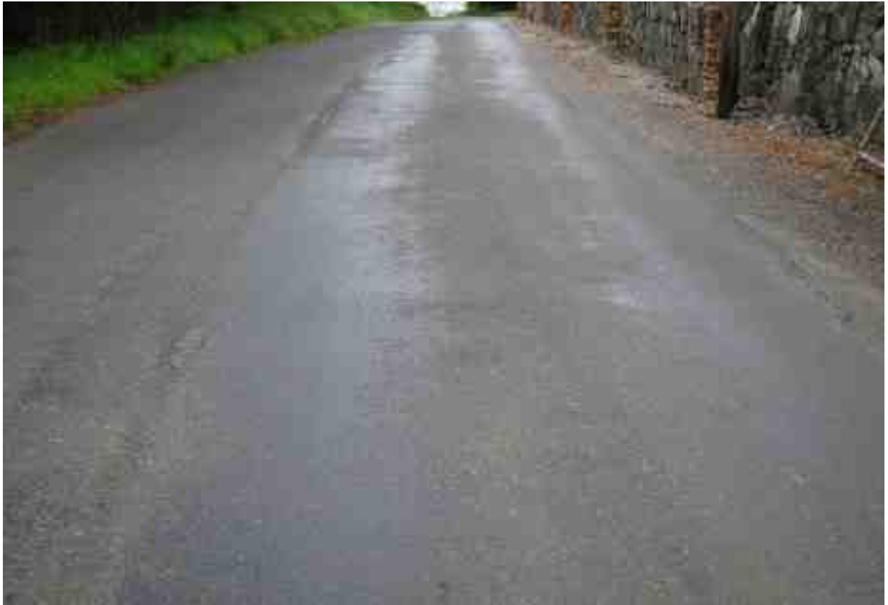
Bleeding. Dark, shiny areas show where binder has worked to surface.
