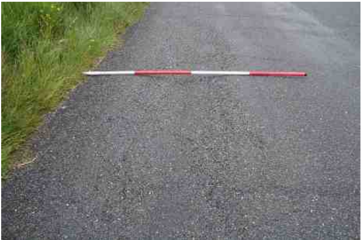
Severe Rutting caused by poor base or subgrade problems.
