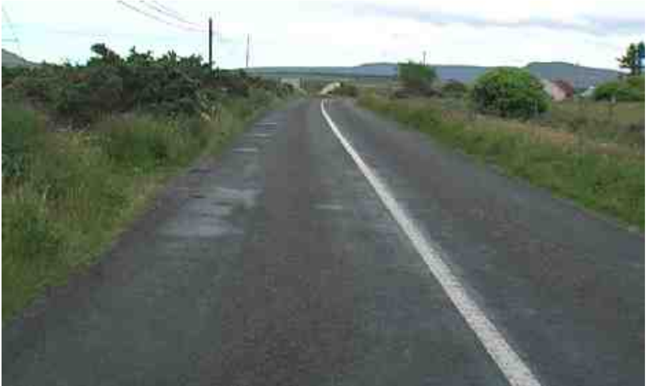
Rating 4: Rutting, potholes and patching in wheelpath. Structural distresses are clear.
