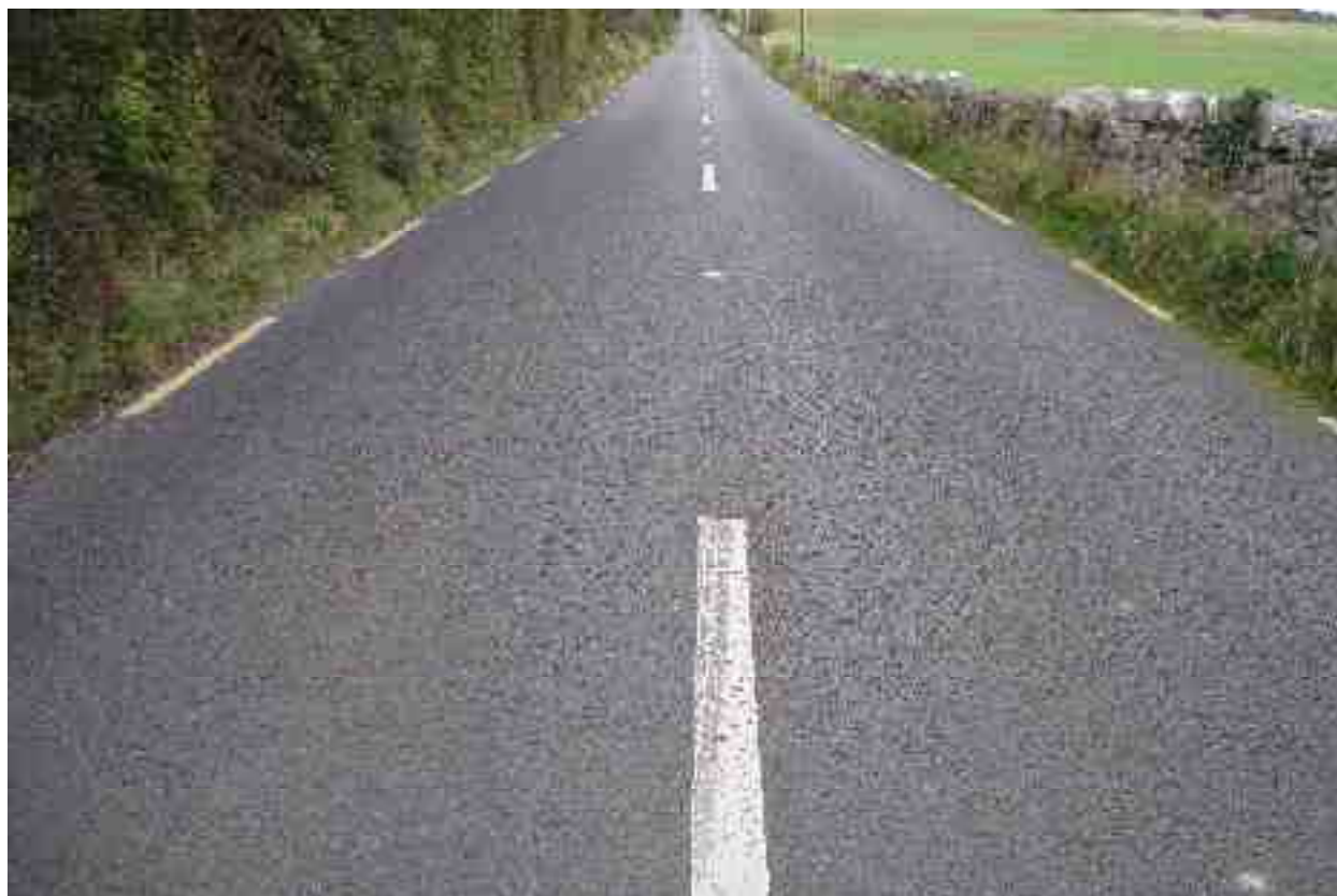
Rating 10: Road with no visible pavement defects.
