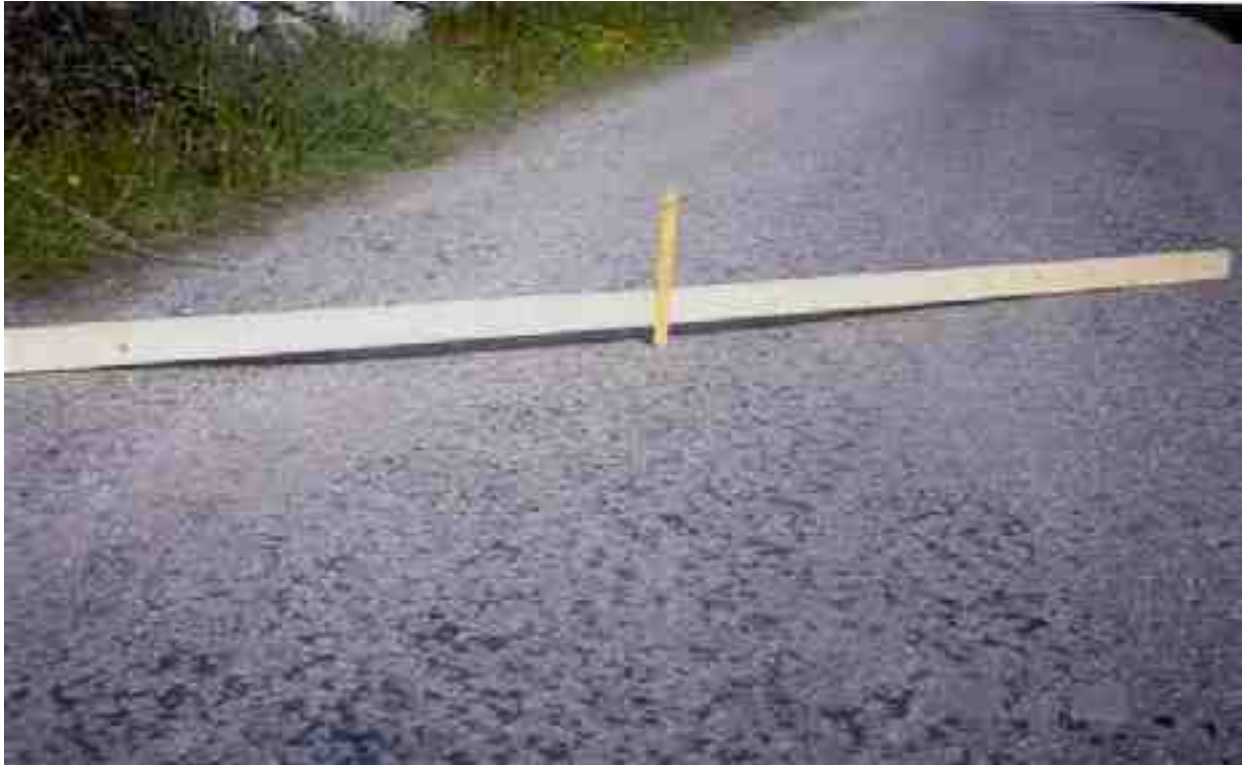
Significant depression visible in concentrated area.
