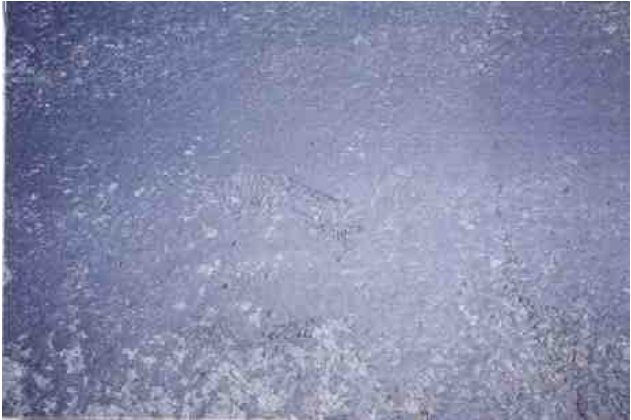
Bleeding/Fatting-up of binder needs repair.
