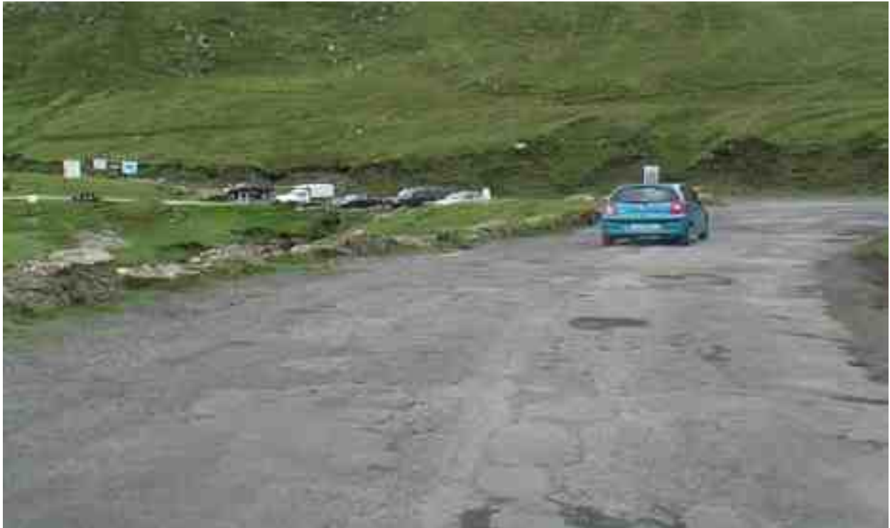
Rating 2: Severely deteriorated, extensive patching and structural problems , loss of surfacing in places.
