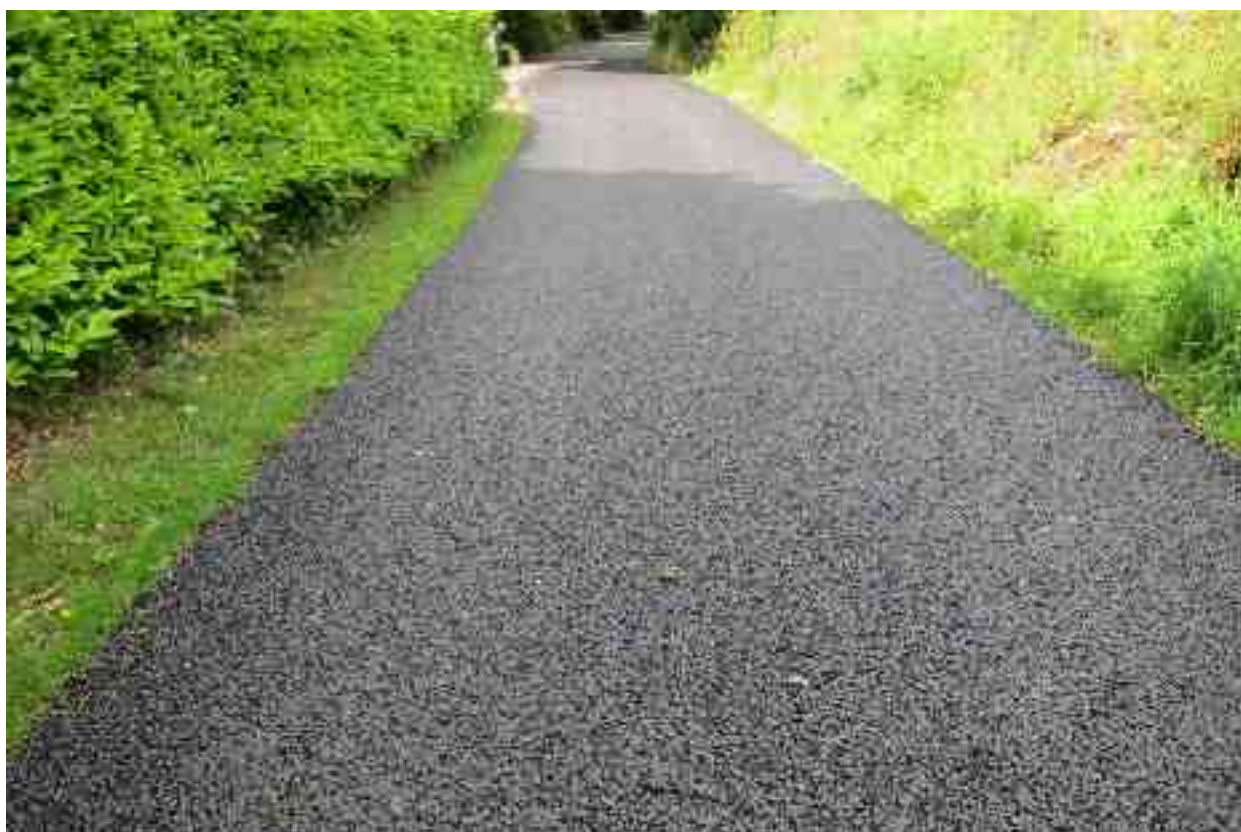
Rating 10: New overlay, local road, no defects.
