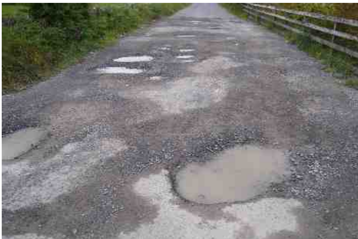
Rating 1: Significant loss of pavement surface, Large quantities of severe potholes.
