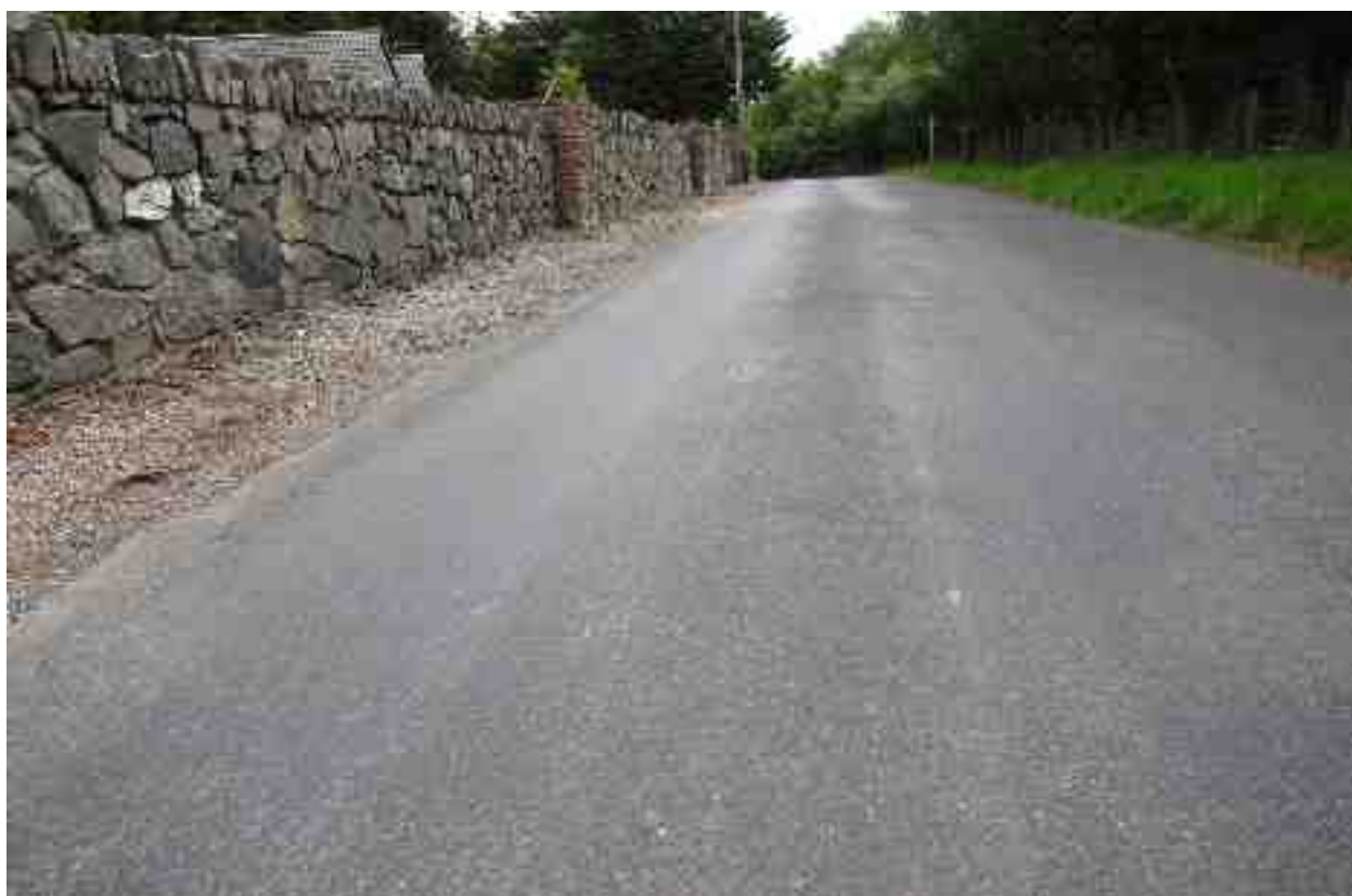
Rating 8: Significant Bleeding, 10% to 30% of surface, note shine off dry road.
