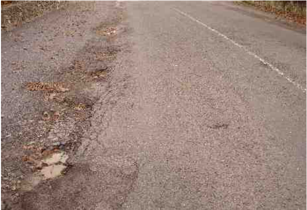
Edge Breakup at the edge of the road pavement.
