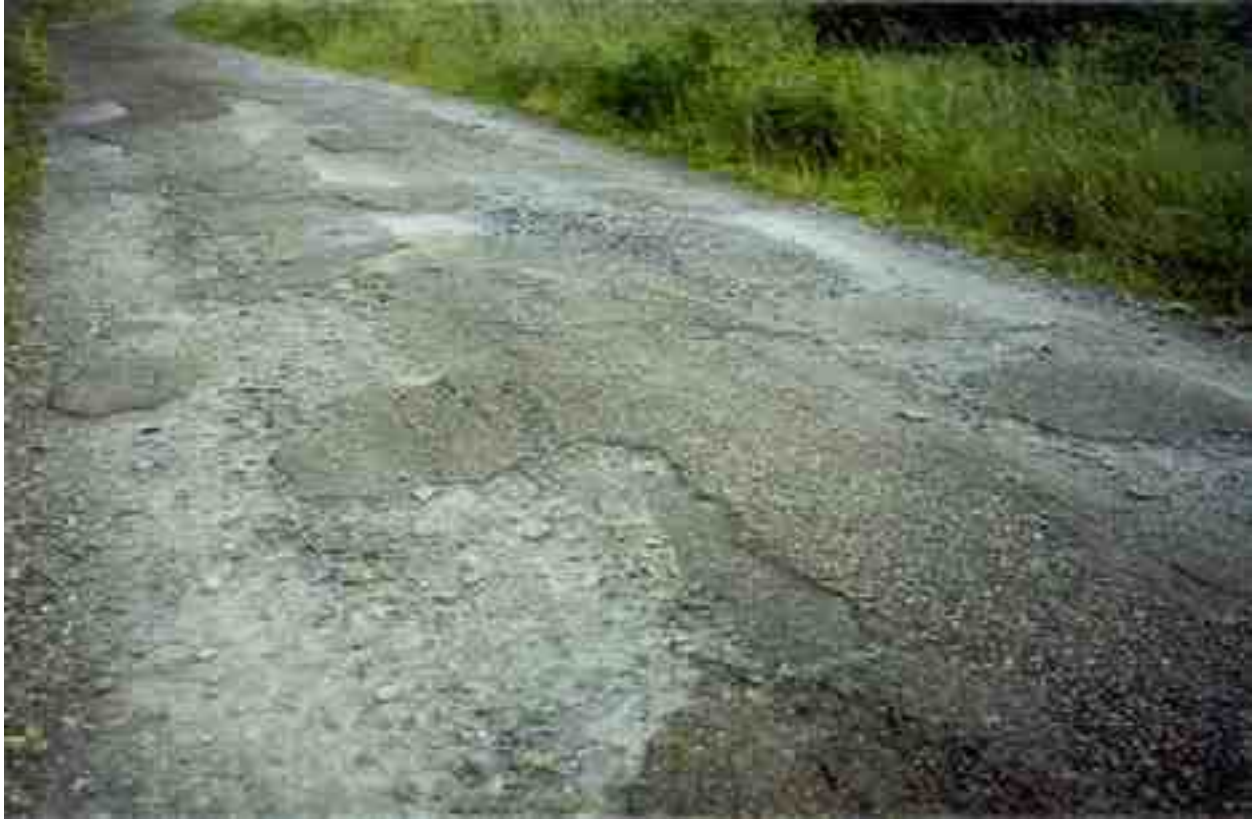
Rating 1: Entire width of road disintegrated with reconstruction required.
