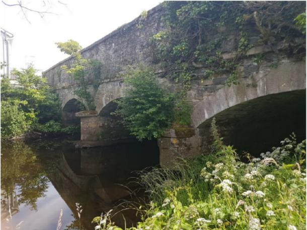
Bridge requiring scour protection and general maintenance work
